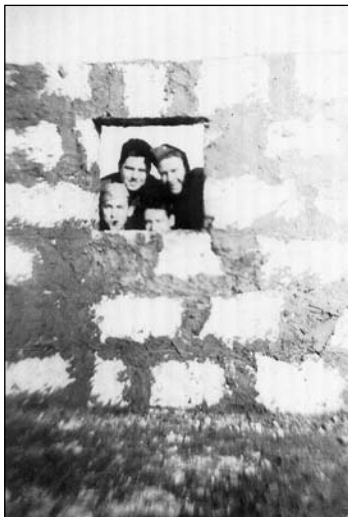
Peering through a window of the half-built Tuffa wall for the enlisted men's tent. Cleon is in the upper right.
